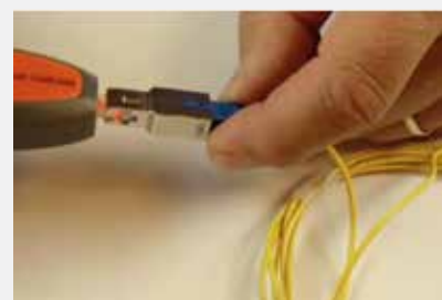
Check the termination
