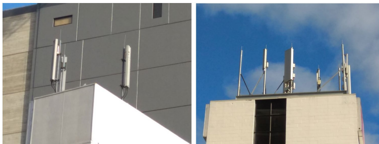
Figure 6–9 Rooftop mounted deployments
