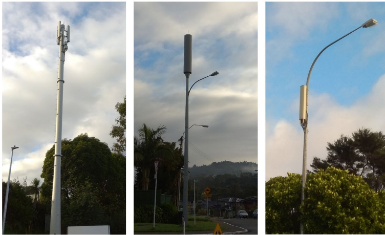
Figure 6–8 Tower/pole-mounted deployments (standalone mobile tower, top/side of lamp post)
